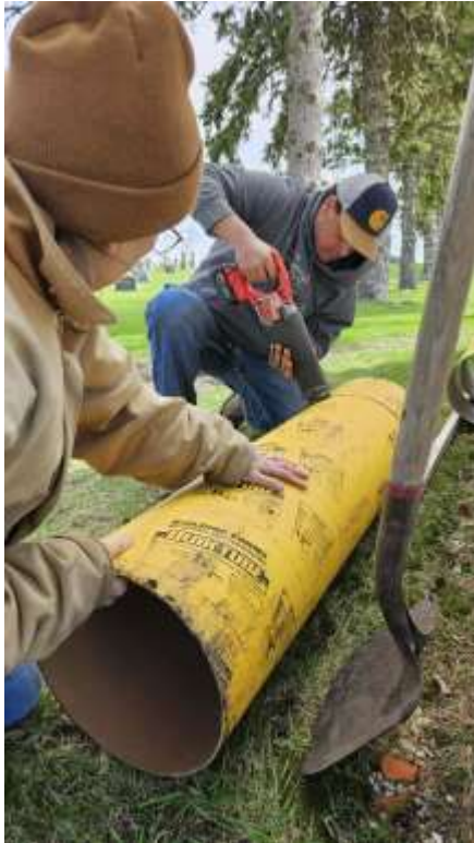
Zachary Zeleke preparing a concrete form for base for the base of the Information Board.
